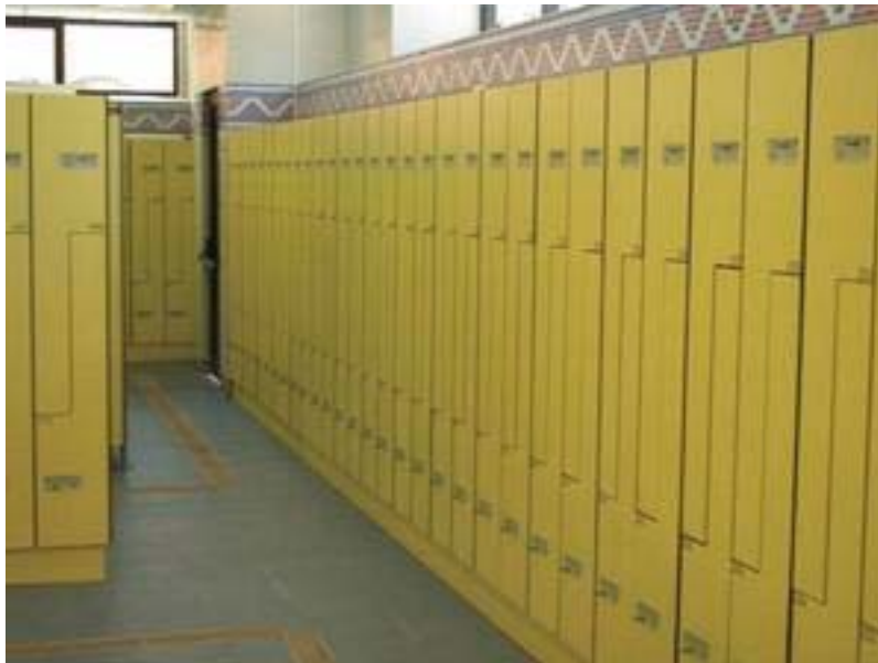
This photo was taken in a locker room, where card Kimaldi Ndcan 16R was installed.
